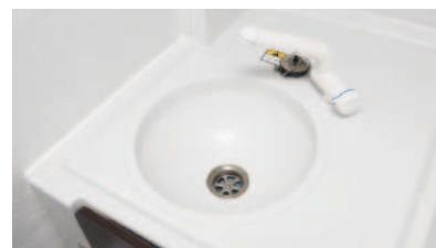
Sink (Rest room)
