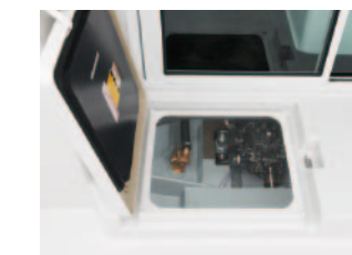
Engine room entrance hatch [Aft]
